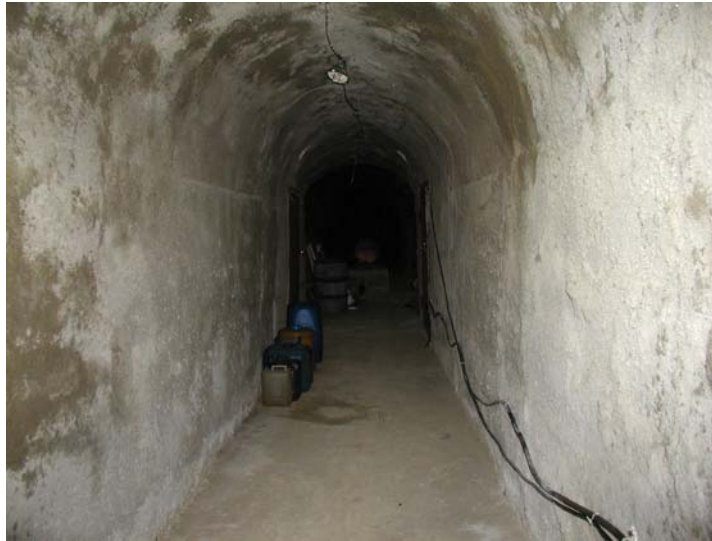
Photo. 1 Georgian Seismic Network. Tunnel leading to quiet vault for seismometer.
