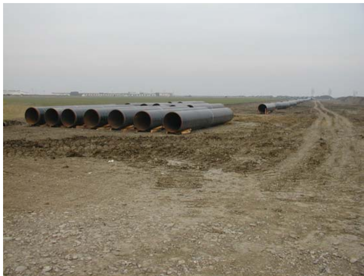
Photo. 3 Construction of oil pipeline. Local earthquakes monitored by developing seismic networks.
