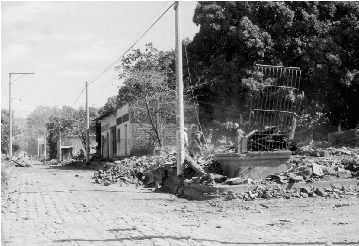
Fig. 21. Collapsed adobe house in San Agustín, of which only the door remains standing after the 13 January earthquake; behind are houses of mixto and lamina , which have survived the earthquake.
