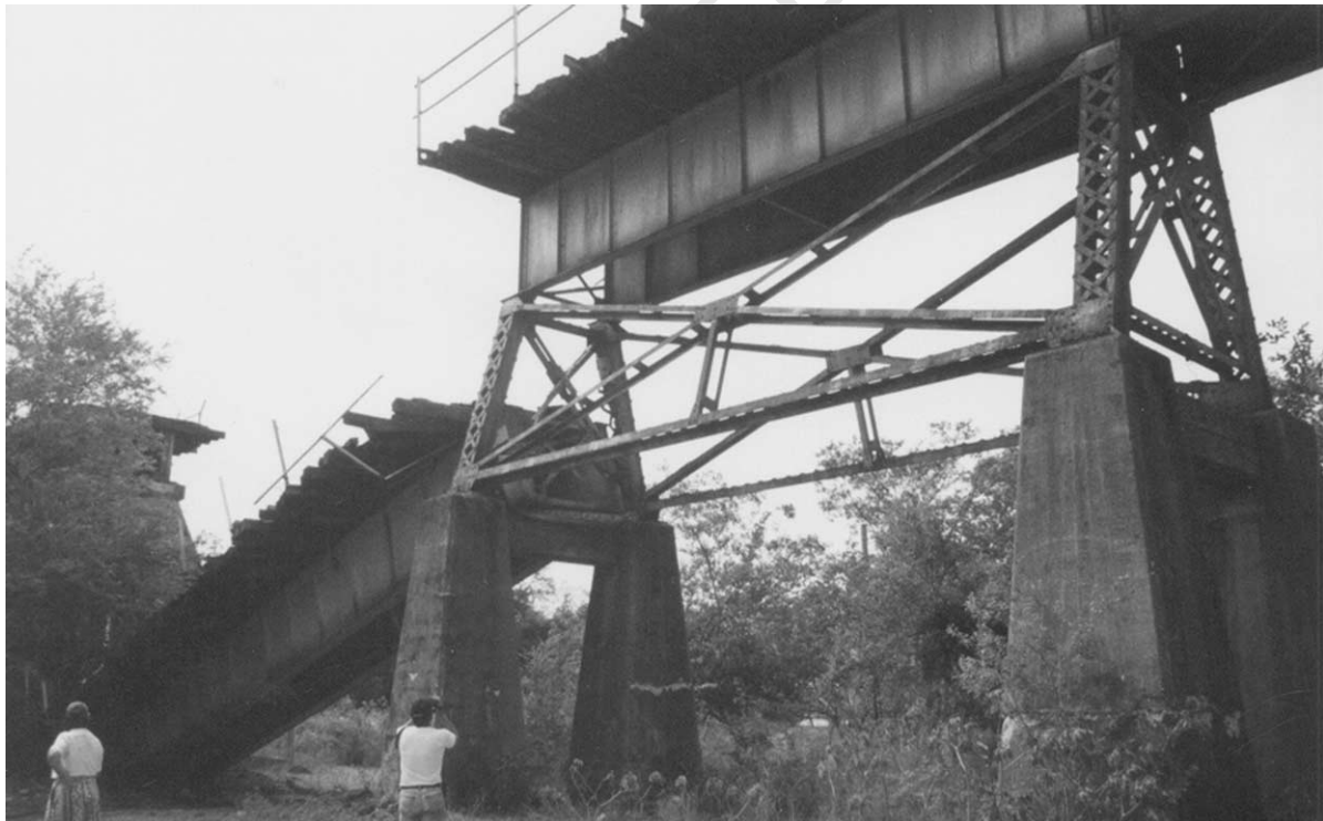
Fig. 20. Collapse of railway bridge due to lateral spreading on banks of the Lempa River.
