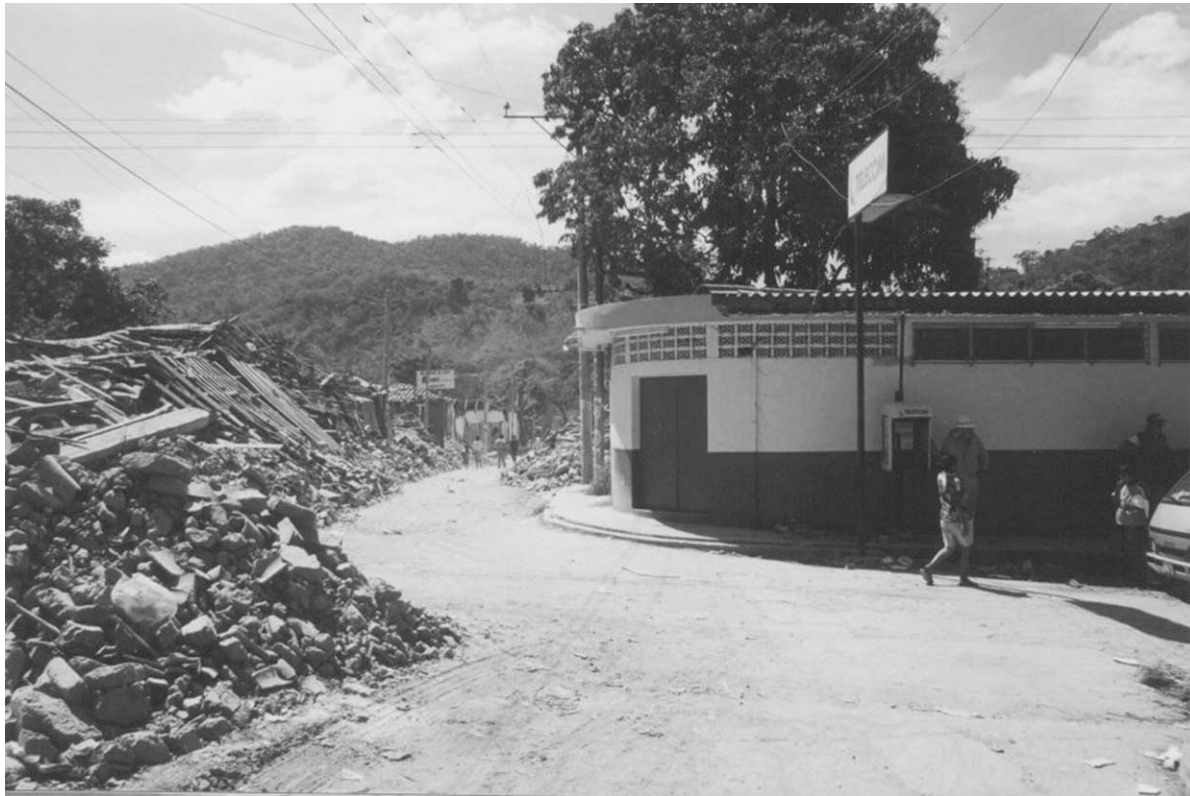
Fig. 22. Guadalupe following the 13 February earthquake, contrasting total collapse of adobe houses with the almost undamaged state of the reinforced masonry building to the right.
