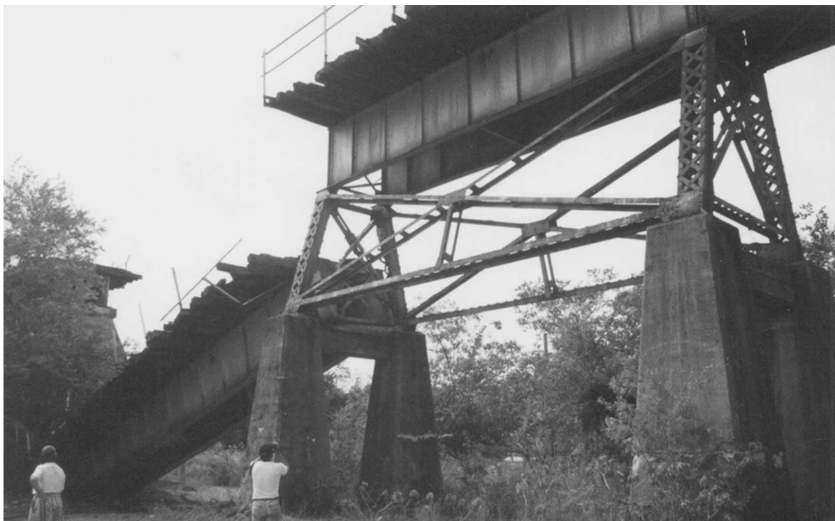
Fig. 20. Collapse of railway bridge due to lateral spreading on banks of the Lempa River.
