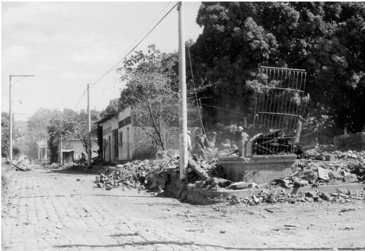
Fig. 21. Collapsed adobe house in San Agustín, of which only the door remains standing after the 13 January earthquake; behind are houses of mixto and lamina , which have survived the earthquake.
