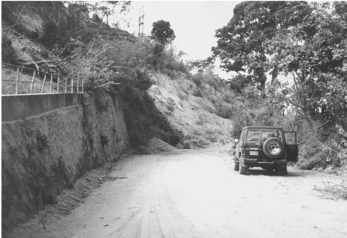
Fig. 15. Debris fall from the tierra blanca near Comasagua.
