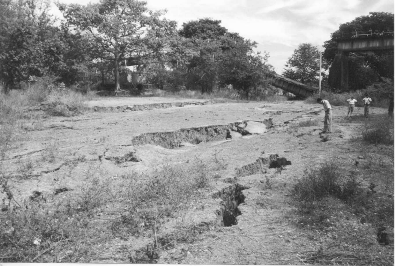
Fig. 19. Lateral spreading on river bank at San Nicolas Lempa.
